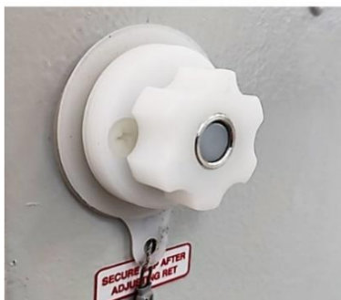
Engaged with internal RET Motor position
