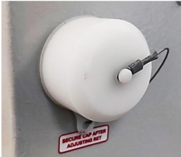
Unscrew/Screw the cap for tilt adjustment process
