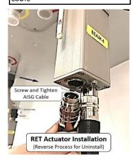
Step 8: RET Actuator installation complete.
